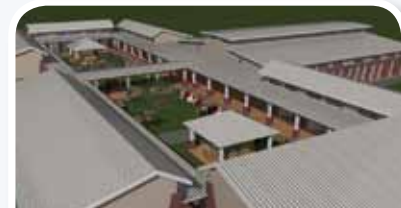
Catherine Booth Hospital - MDR TB Isolation Facility
