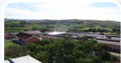
Catherine Booth Hospital - MDR TB Isolation Facility
