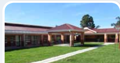
Catherine Booth Hospital - MDR TB Isolation Facility
