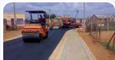
20T Roads and Stormwater Programme rolled out in Mohlakeng, West Rand
