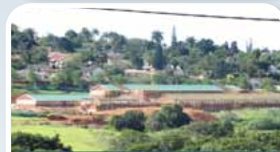
Empangeni Rail High School
